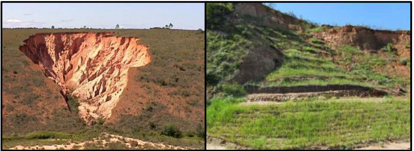
Figure 12: Vetiver System Erosion Control (Before and After). © Paul Truong
