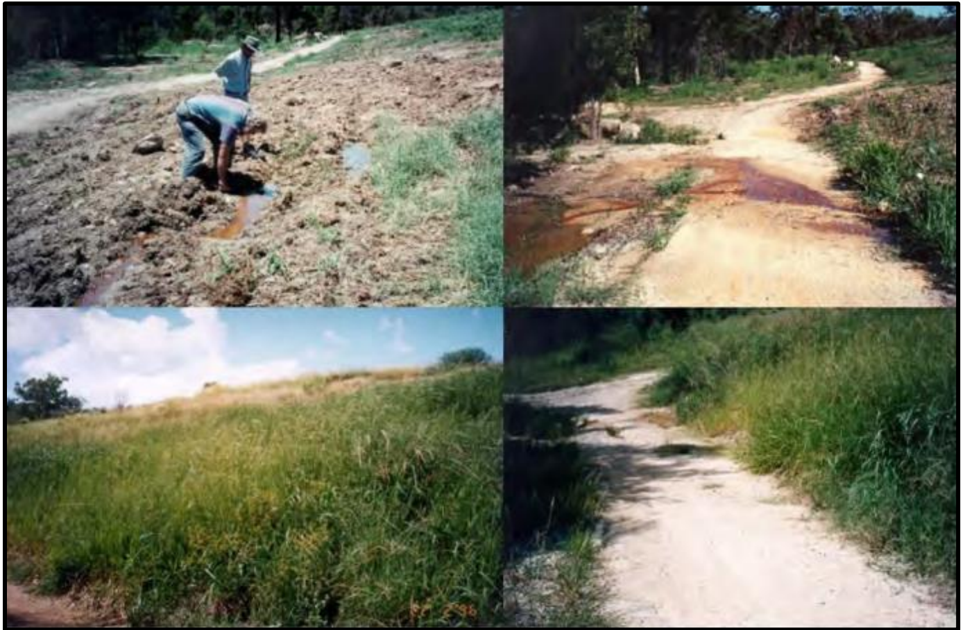
Figure 9: Guangdong Province (China). Vetiver System Used to Control Leachate seepage from closed landfill. Before (Top), After (Bottom). © Paul Truong
