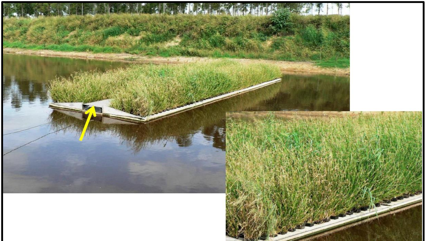
Figure 10: Australia: Industrial Wastewater Treatment Using Vetiver Floating Pontoons
