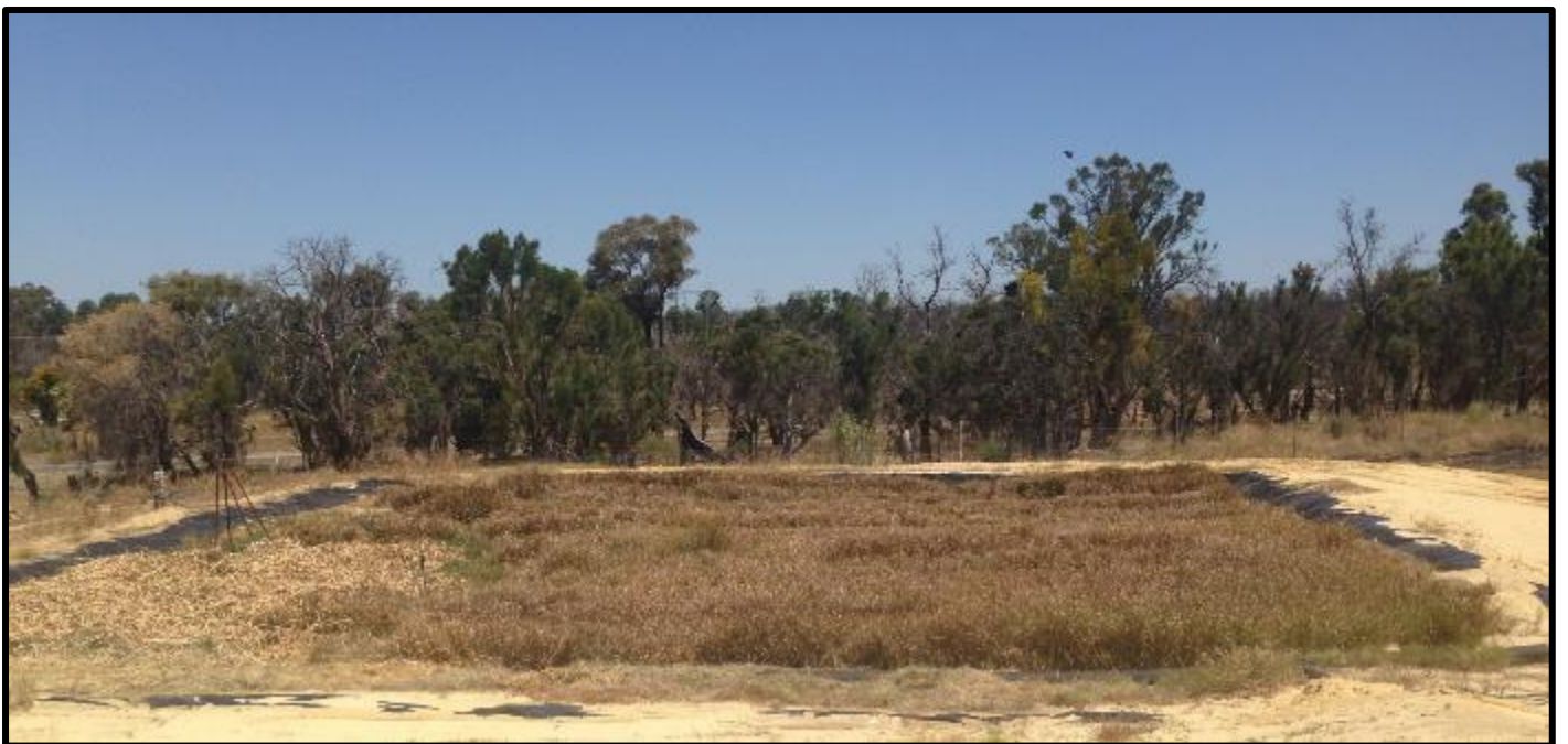
Figure 6: Shire of Waroona (WA) Septic Treatment Plant Vetiver System (Subsurface "Flood and Drain" Irrigation). At the time of this photo the system was being operated poorly – hence dried out VG failing to function effectively.
