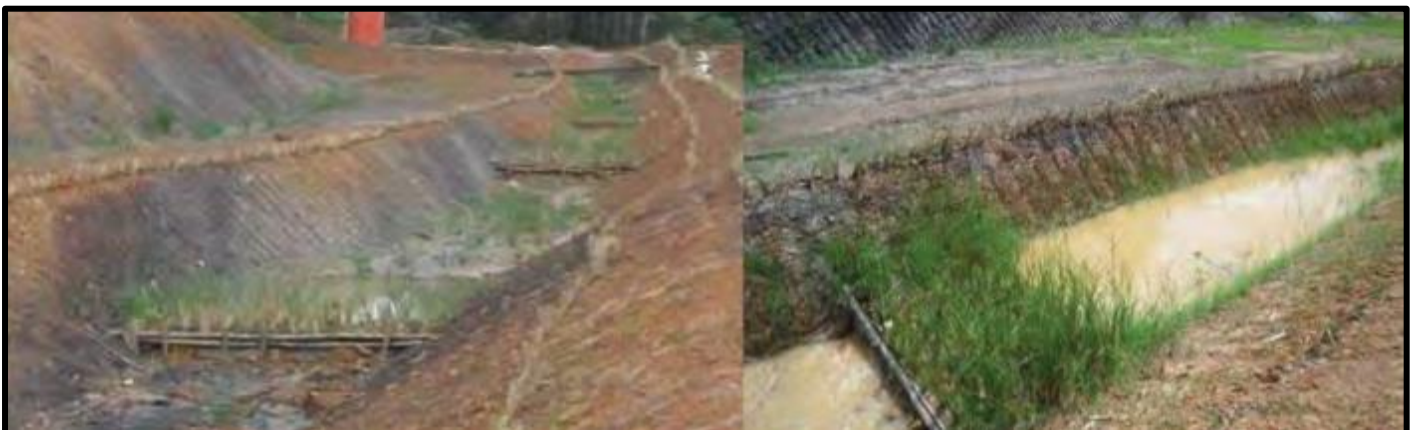
Figure 13: Vetiver System used for Sediment Traps (cross-channel), and Bank Stabilization (along channel banks). © Paul Truong Simeon Kendall
