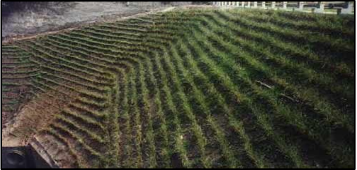
Figure 11: Vetiver System Dam Construction may provide significant financial and environmental benefits over more typical hard concrete engineering. © Paul Truong
