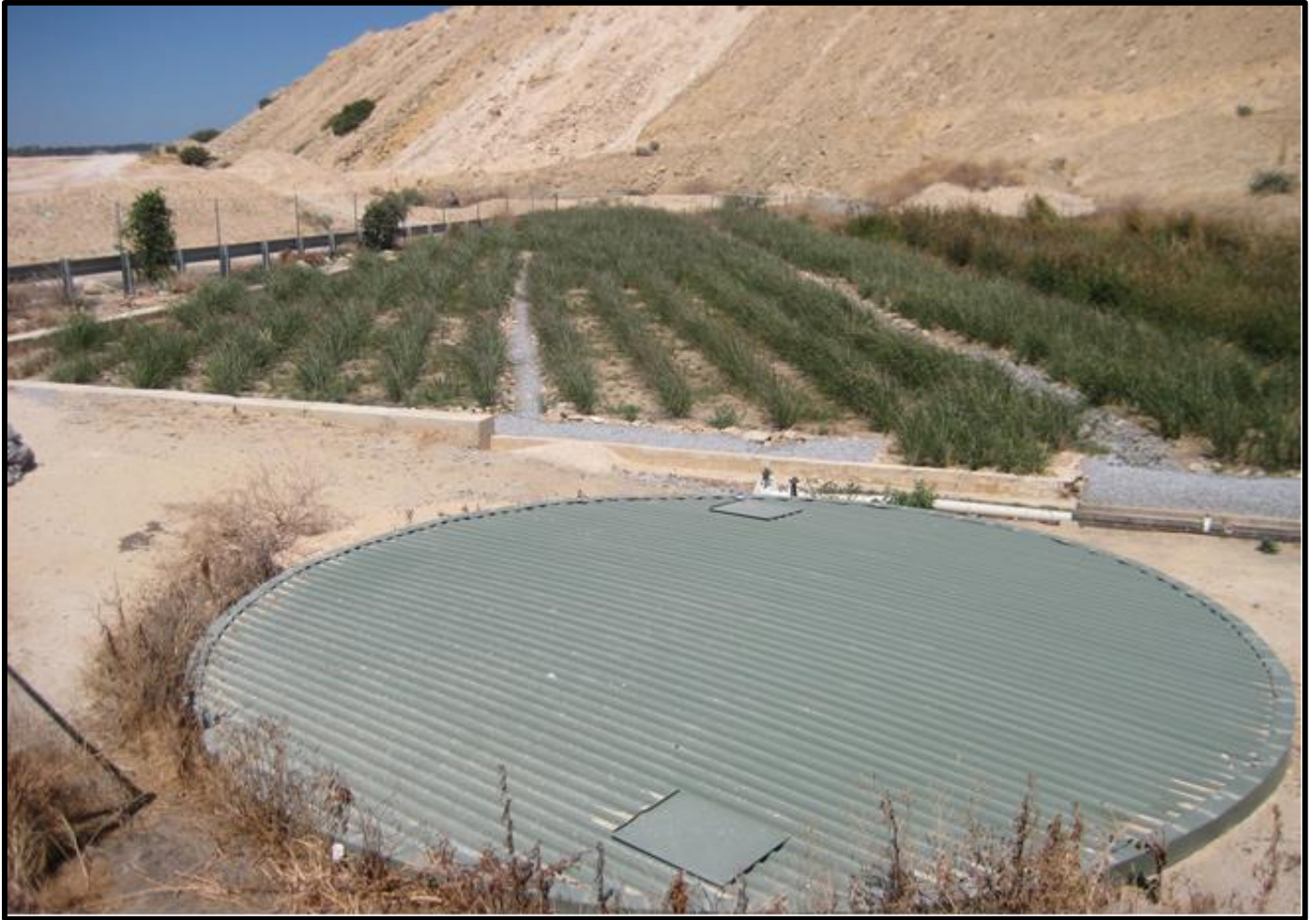
Figure 5: MRC (WA) Truck Wash Effluent Vetiver System (Sub-surface Flow) – Approximately 3 Months Growth from VG slips
