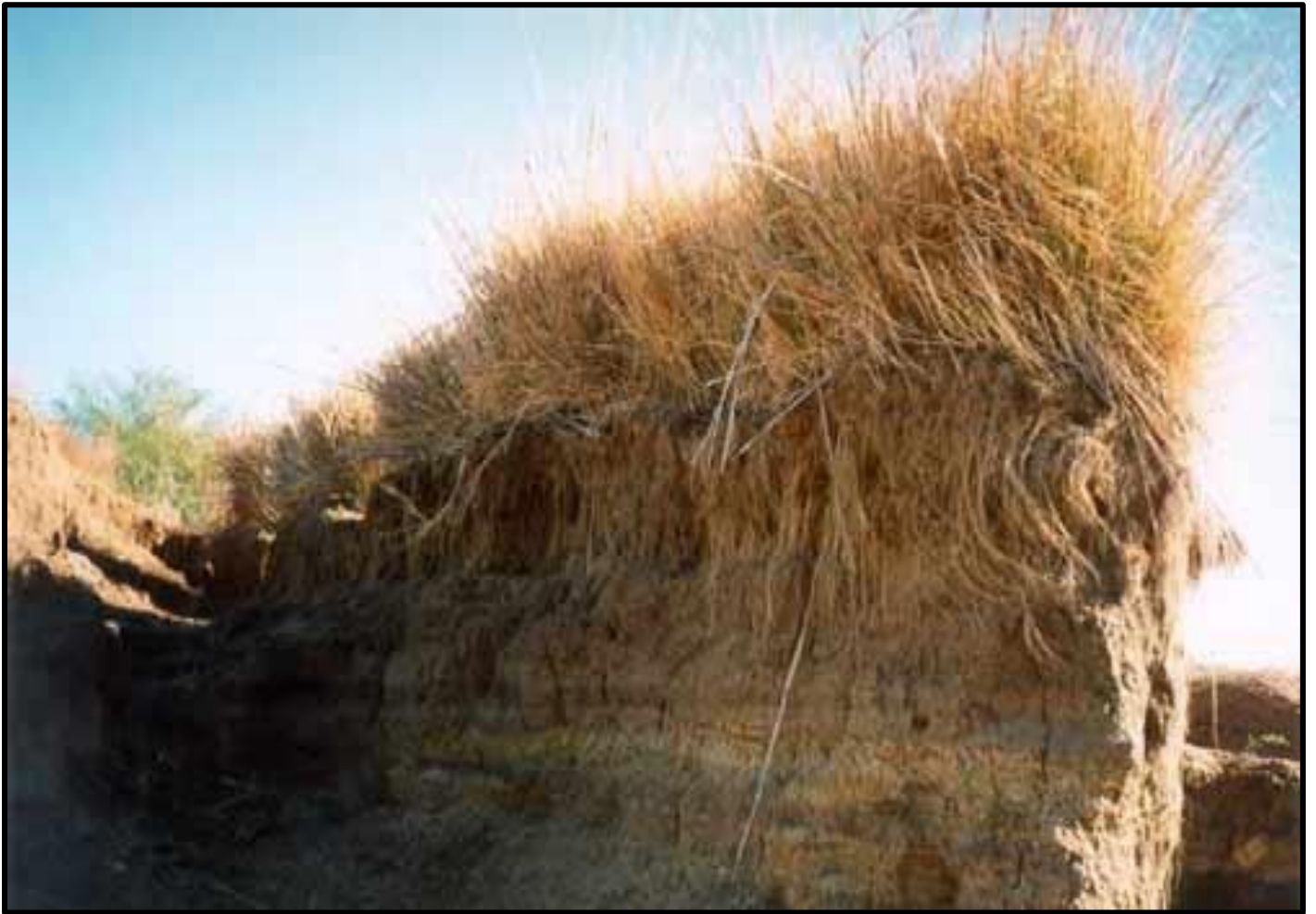
Figure 14: Vetiver System Roots Held up this Wall against Active Erosion © Paul Truong
